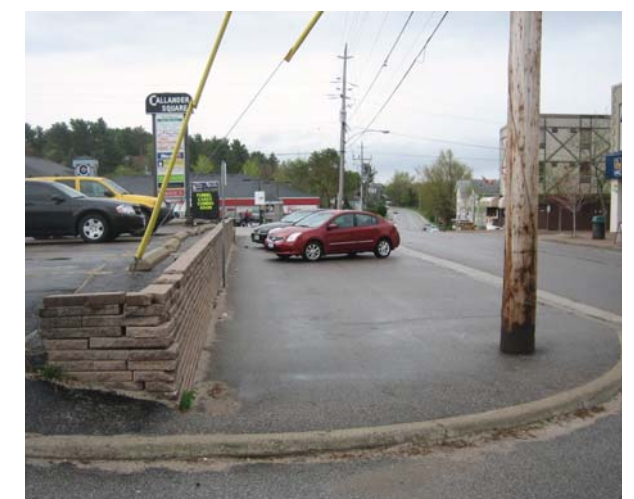
Current Condition of North East Corner of Main and Lansdowne Streets
