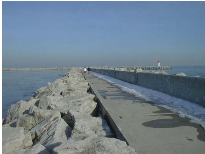
Figure 4. Concrete walkway with parapet wall on breakwater (Baird, 2008)
