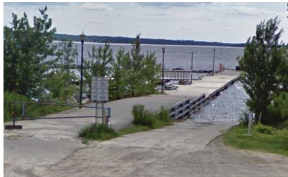
Current Conditions of Waterfront Pier and Marina
